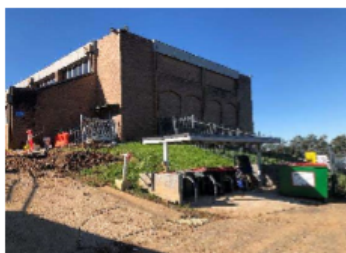
Figure 15: External view of Block C, facing north from within the campus. (Source: NBRS)
