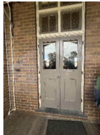
Figure 39: Proposed door to be replaced due to accessibility non-compliance. Note that the existing door frame and fanlights would be retained (Source: NBRS).
