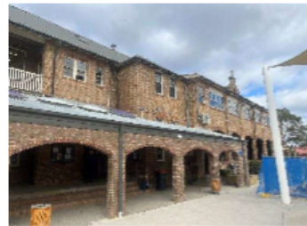
Figure 7: External view of the western façade of the Block A. (Source: NBRS).
