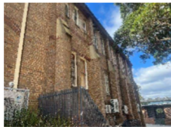
Figure 8: External view of the southern façade of the Block A. (Source: NBRS).
