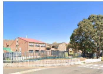
Figure 19: External view of Block F, facing southeast from Marie Street. Notably the building largely obscures Block A from Marie Street (Source: Google Streetview).
