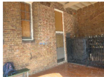
Figure 9: External view of the enclosure and creation of new openings on the western side of the building to facilitate the ongoing use as a class rooms. (Source: NBRS).
