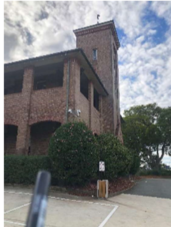
Figure 4: External view of the Romanesque-style façade and tower on the east side of the building. (Source: NBRS).
