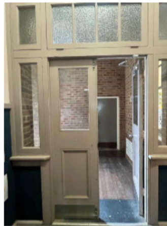
Figure 38: Proposed door to be replaced due to accessibility non-compliance. Note that the existing door frame, sidelights and fanlights would be retained (Source: NBRS).
