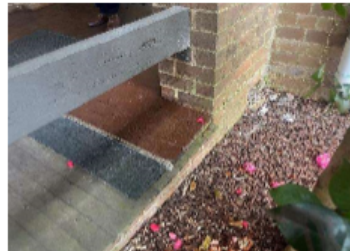
Figure 10: External view of the eastern verandah and the existing performance solutions for disability access. (Source: NBRS)
