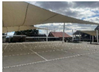
Figure 18: External view of Block F, facing west from in front of Block A. (Source: NBRS).
