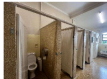
Figure 37: Interior view of first floor existing female bathroom. (Source: NBRS).
