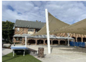
Figure 47: Existing contemporary metal roof of Block B (Source: NBRS).
